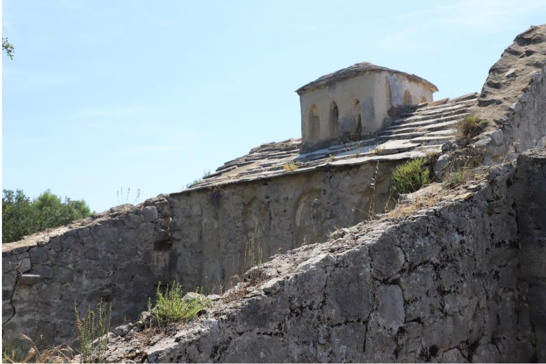
Fig. 26. Church of Saint John the Baptist, Lopud.
