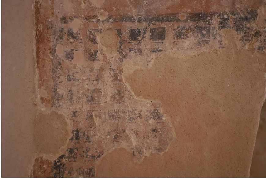
Fig. 112. Church of Saint John the Baptist, Šipan. Eastern blind arch on the south wall. Detail of the ornament.
