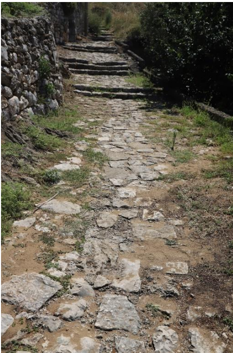
Fig 16. Communal road on Lopud.
