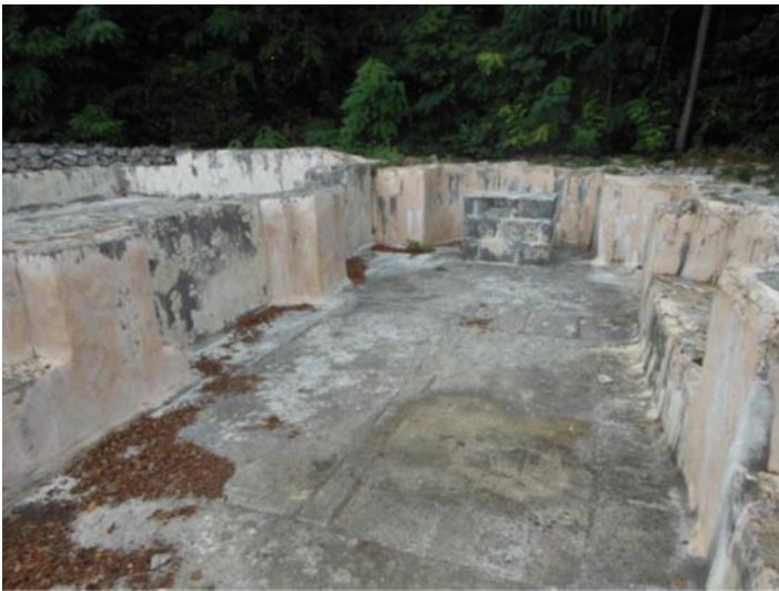
Fig. 39. Church of Saint Michael, Koločep, 11th century. Condition after the reconstruction.
