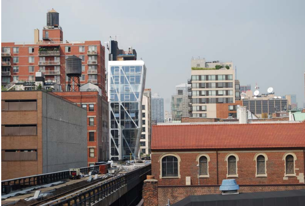
Figure 4.1: HL23 and the High Line Park under construction, July 7, 2010. Photographer: Per-Johan Dahl.
