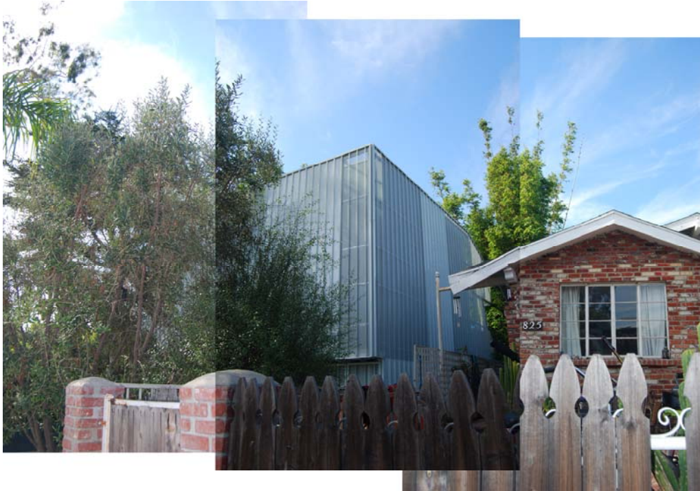
Figure 3.33: The accessory unit at Palms Residence in Venice, CA, October 28, 2011. Collage by Per-Johan Dahl.
