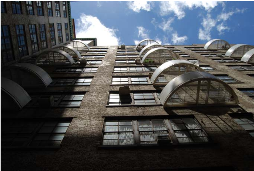
Figure 2.12: The balconies of Westbeth as a second means of egress. Photography: Per-Johan Dahl.
