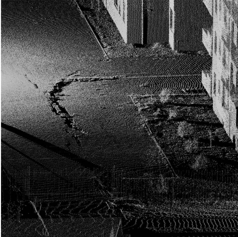
Figure B.16. LiDAR photography for Riesco Building from Kayen (2016), personal communication.
