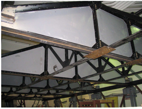
Figure 14: The Ceiling Structure
