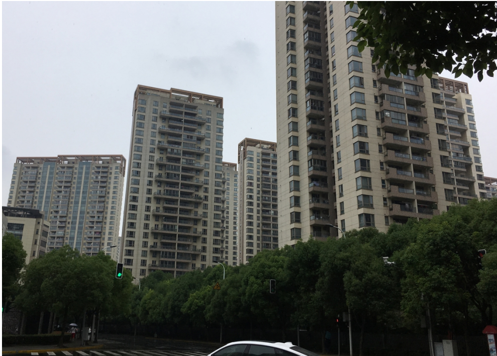
Figure 4 Lianyang Biyun Community in Pudong. Photo by author in June,2017.
