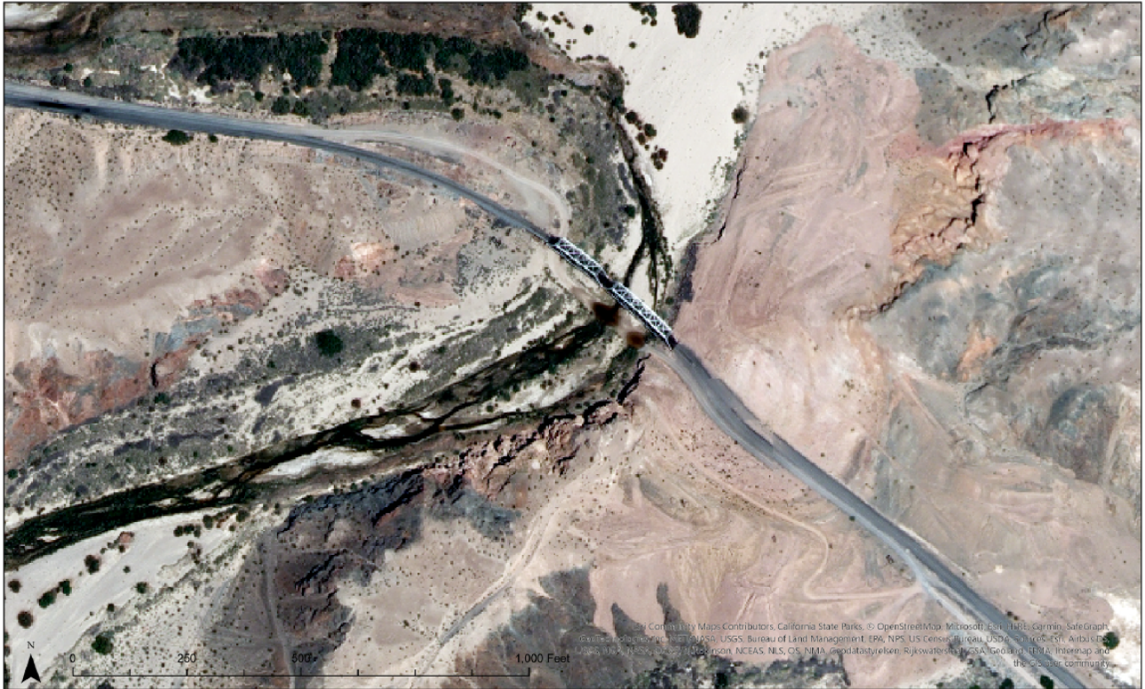
Figure 13. Aerial Satellite Imagery of Afton Canyon at Mojave River Deep Crossing, 26 April 2010.
