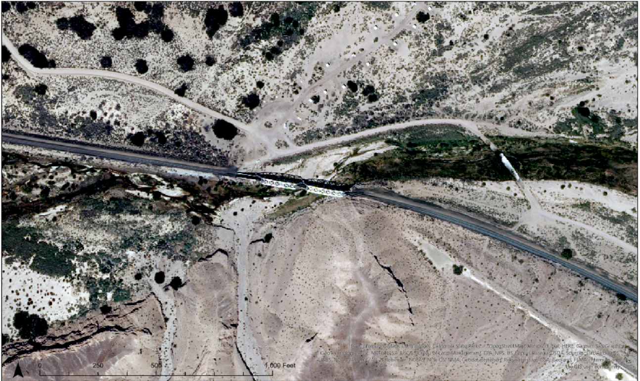
Figure 9. Aerial Satellite Imagery of Afton Canyon at Union Pacific Railway Bridge. 26 April 2010.
