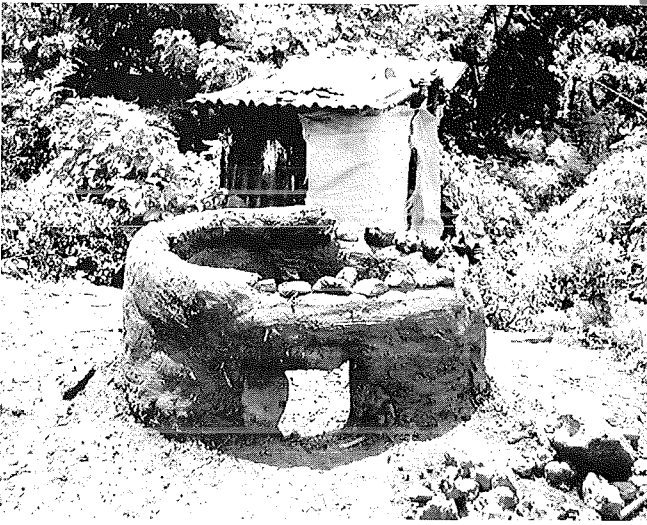
Figure 4.1 Ceramic kiln under construction, San Isidro Texcaltitan, Veracruz. Photograph by Elizabeth A. Hoag
