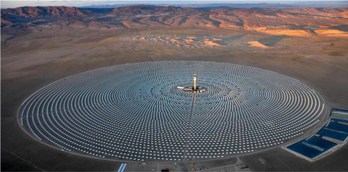
Figure 2: Crescent Dunes Solar Energy Project in Tonopah, Nevada (source: SolarReserve.com)
