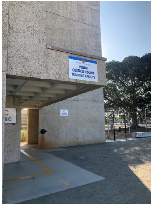
Figure 5.1: Exterior shot of Building C, one of the many structures that house classrooms at the San Diego Regional Public Safety Training Institute. A sign on the concrete façade reads “The City of San Diego Police Obstacle Course Training Facility,” San Diego, California, November 4, 2019 (photo credit: Christina Aushana)
