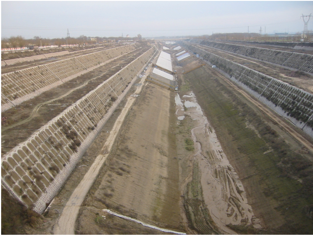
Figure 1.2- SNWTP Middle Route Canal Under Construction
