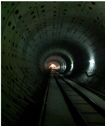
Figure 1.4- Inside the SNWTP Yellow River Tunnel (pre-inundation)
