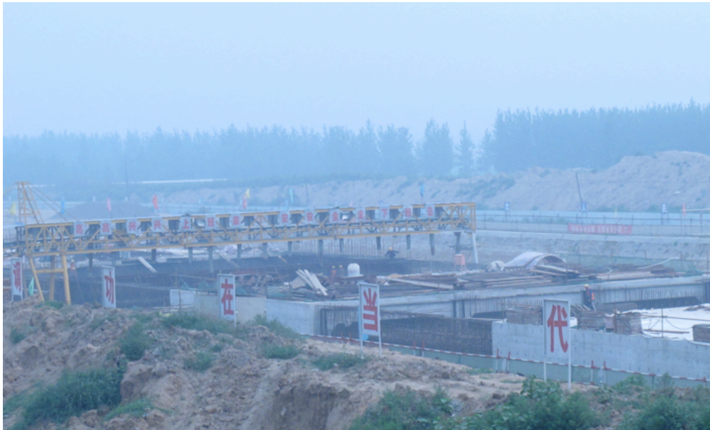
Figure 5.1- MR Canal Under Construction in Hebei
