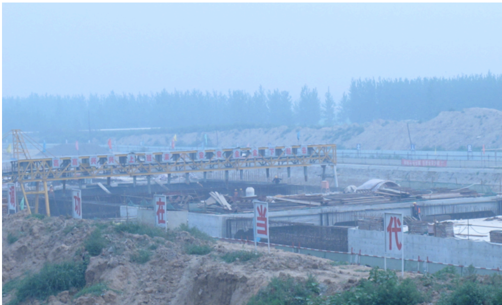
Figure 5.1- MR Canal Under Construction in Hebei
