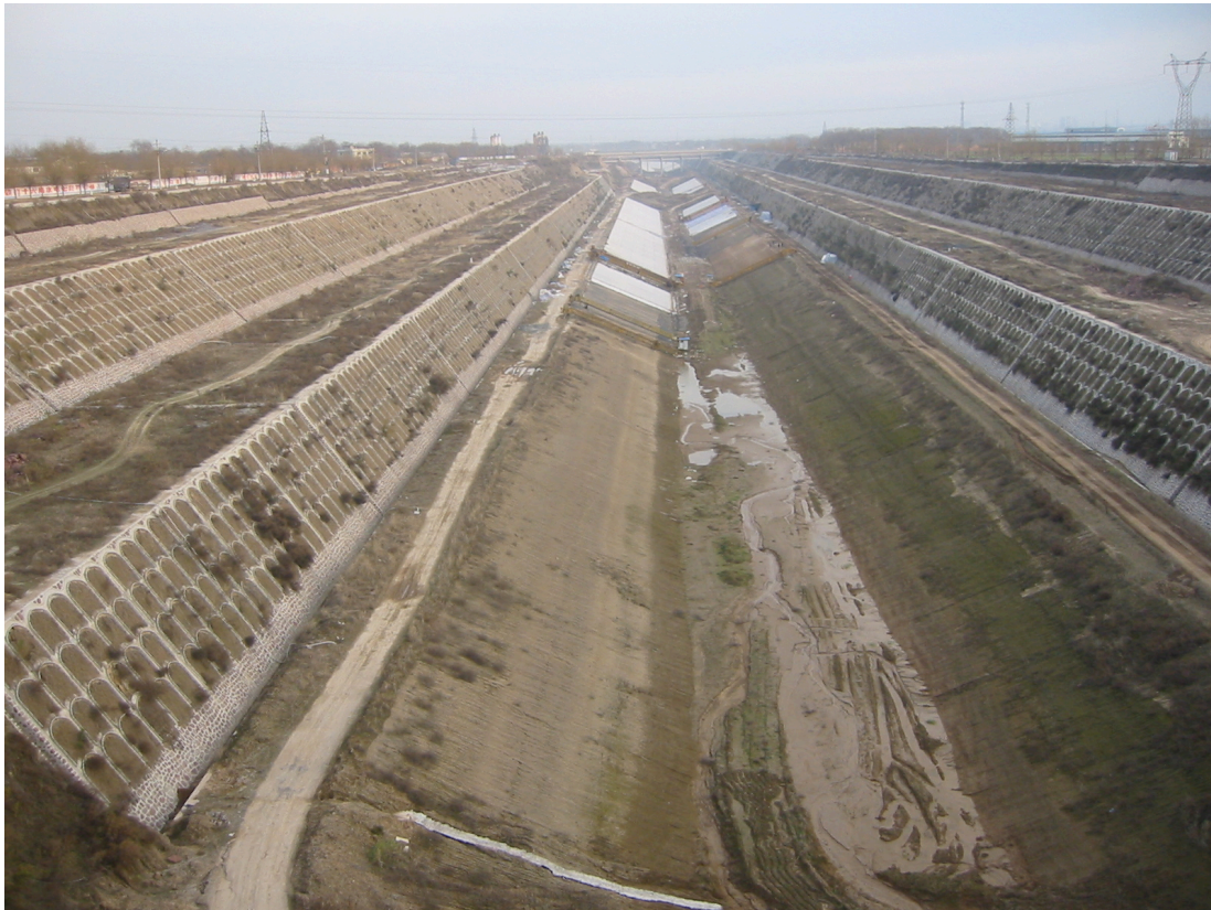
Figure 1.2- SNWTP Middle Route Canal Under Construction
