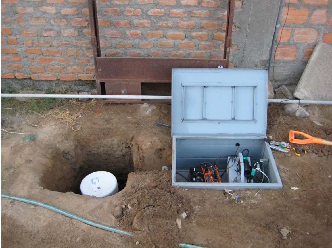
Figure 5.2 – Seismic station installation in Peru
