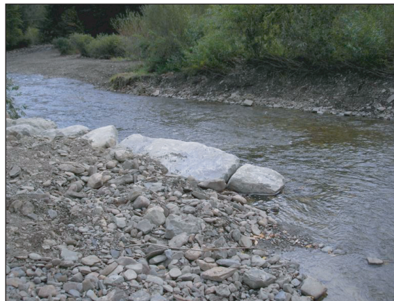
Figure 12. One of the rock vanes built on the north bank of Canasawacta Creek. The photo was taken looking downstream.
