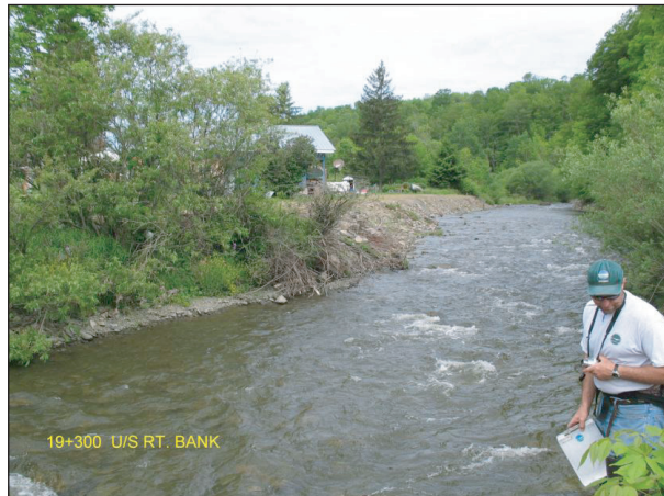
Figure 3. Looking upstream from the bridge at Moon Hill Road. The bridge is just out of the picture to the left. One of the houses located between Route 23 and Cansawacta Creek can be seen in the center of the photo.
