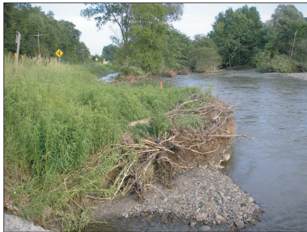
Figure 7. This photo was taken just upstream from the rip-rap shown in Figure 6 after the June flooding. The creek has cut a new channel closer to Route 23. The vegetation blocks a clear view of the road but the location of Route 23 can be surmised by guide rail and highway sign.
