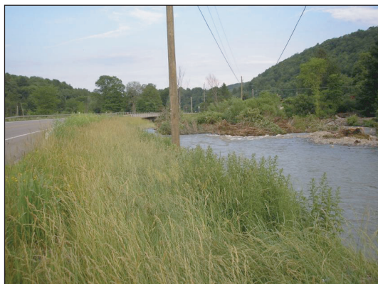
Figure 10. Looking downstream just above the Chan Aldridge bridge (same location as figure 9) just after the June 2006 flood. The utility pole is now on the bank of the creek.
