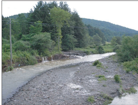
Figure 11. South side of Canasawacta Creek looking upstream from the Chan Aldridge bridge after the June 2006 flooding.
