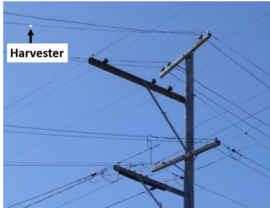
Figure 1.2: Hypothetical energy harvester (to scale) attached to an overhead power distribution line
