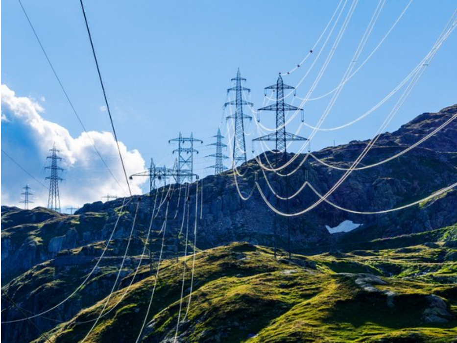
Figure 2.5: Power line sag[3]
