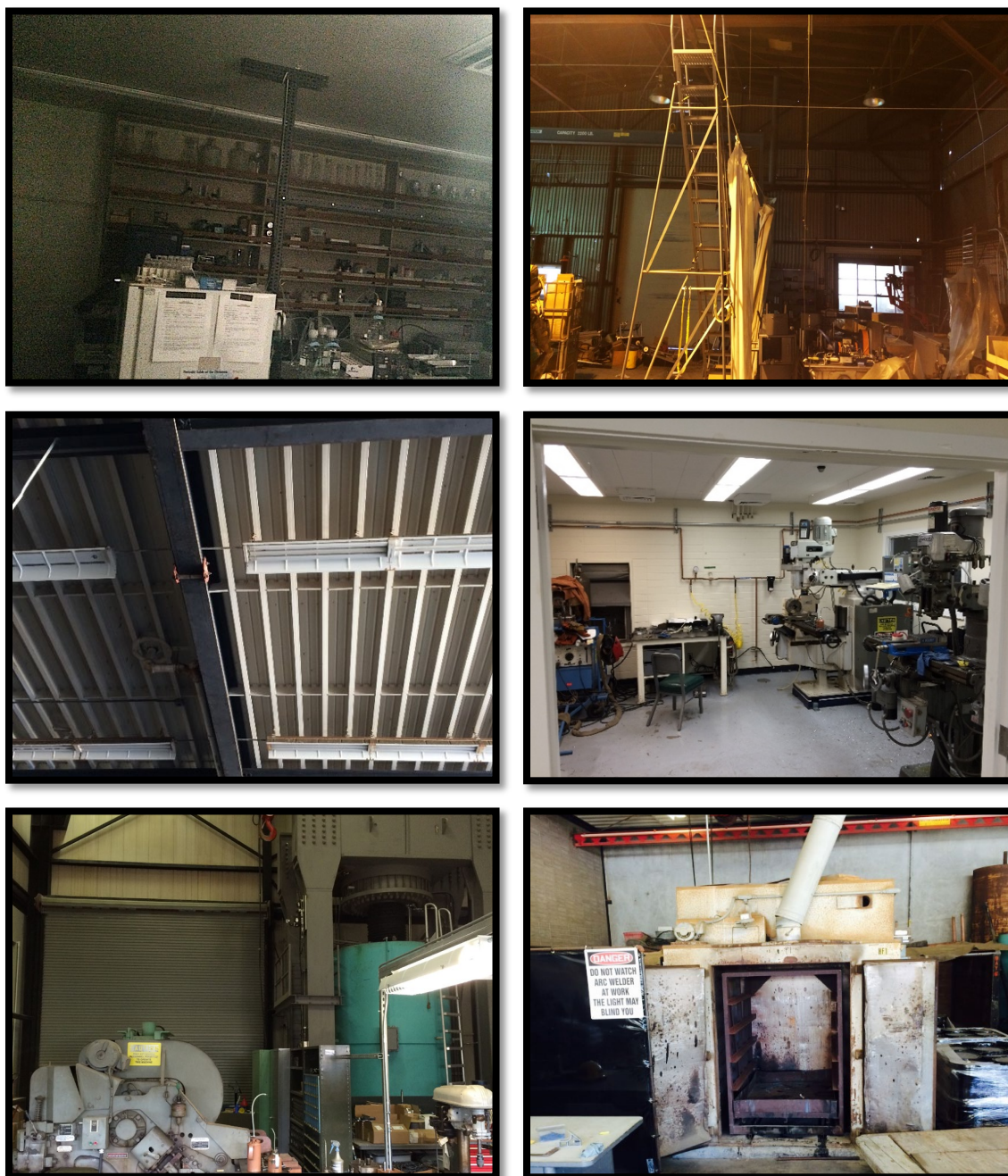
Figure 4.4: Noteworthy characteristics of light industrial buildings. (top left) Lab in Bldg. 154 where a properly licensed and stored ^{137}\text{Cs} source was detected. Its presence was not revealed prior to our measurements. (top right) Interior view of Bldg. 158 high-bay with I-beam support structure and corrugated metal walls. (middle left) Interior view of Bldg. 486 roofing depicting steel roof decking supported by an I-beam structure. (middle right) Interior view of Bldg. 486 with concrete walls and machining equipment. (bottom left) Interior view of high-bay in Bldg. 486 with machining equipment and large rock crusher. (bottom right) Interior view of Bldg. 486 large furnace and welding equipment. Source: personal photographs.
