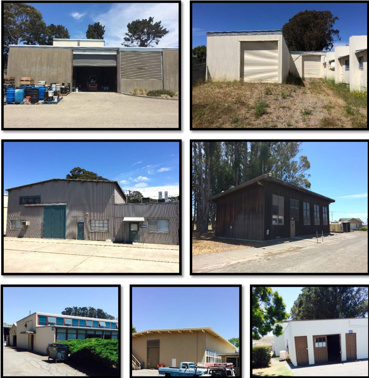
Figure 4.3 Representative light industrial buildings found at Richmond Field Station. (top left) Bldg. 486 contained tilt-up concrete exterior walls, internal cinder block masonry, I-beam structure, and steel roof decking. (top right) Bldg. 128 was built for manufacturing explosive blasting caps; it has areas with concrete walls 2 feet thick as well as corrugated steel walls and an asphalt and wood ceiling over steel trusses. (middle left) Bldg. 158 is a high-bay with an I-beam support structure and corrugated metal walls. (middle right) Bldg. 472 is a unique wooden building used for cutting cross-sections of large trees. (bottom left) Bldg. 480 contained laboratory space for analysis of concrete and asphalt road samples. (bottom middle) Bldg. 478 is a forestry products laboratory and warehouse with climate-controlled spaces. (bottom right) Bldg. 153 is used by mechanical engineering students working on small engines and contains various machining equipment. Source: [98] personal photographs.
