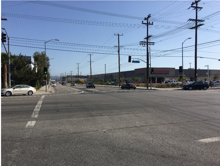
Figure 13 Intersection of Tujunga Avenue and Sherman Way Looking South
