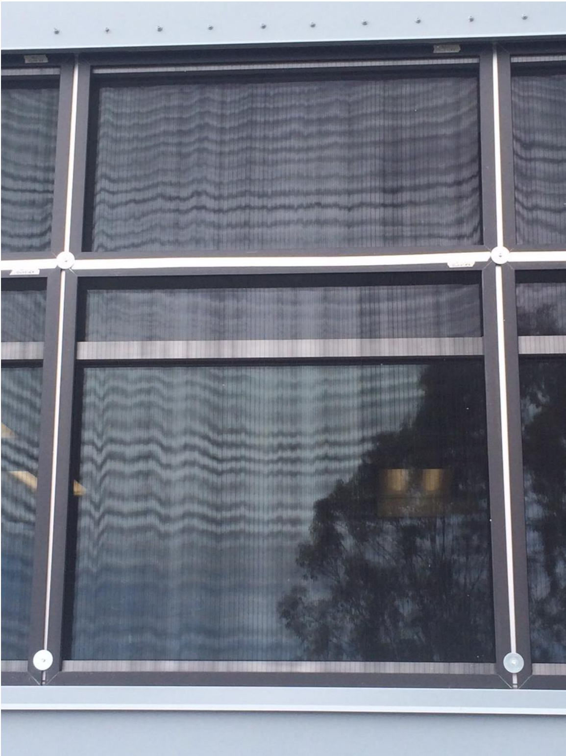
FIGURE 6.13 PHOTOGRAPH OF THE EXTERIOR SHADING S-L SYSTEM FROM THE OUTDOORS.
