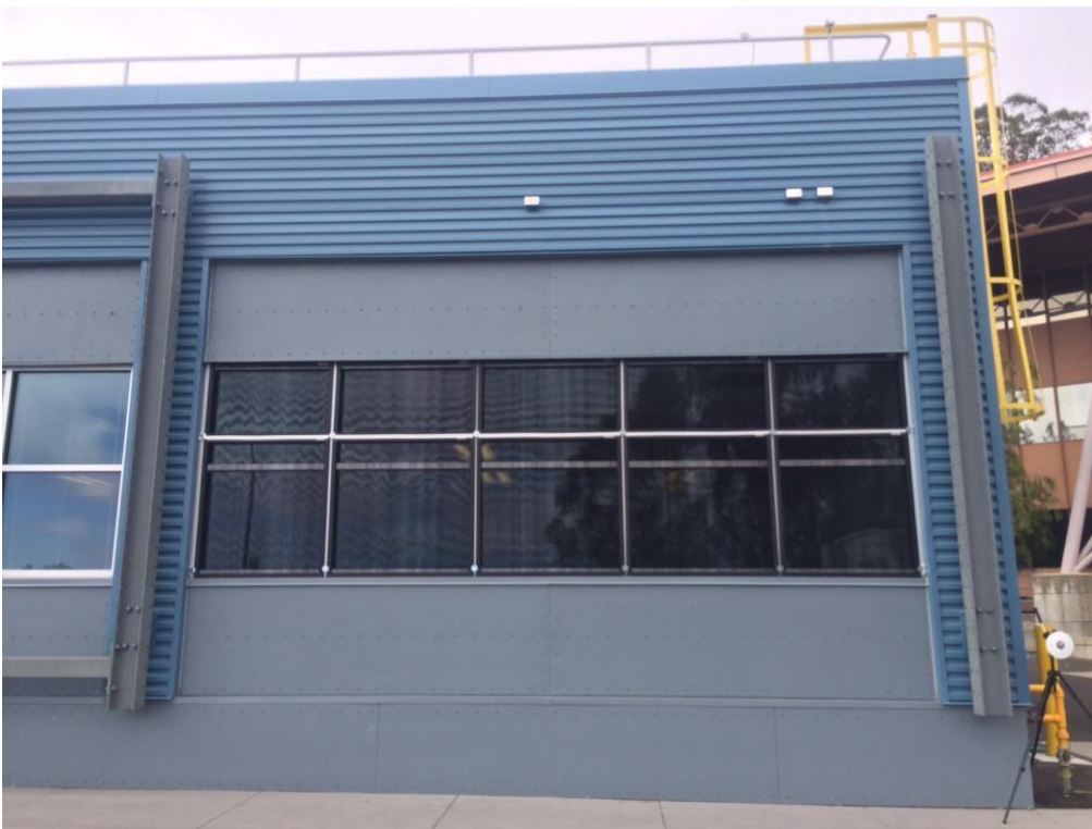
FIGURE 6.12 PHOTOGRAPH OF THE EXTERIOR SHADING S-L SYSTEM FROM THE OUTDOORS
