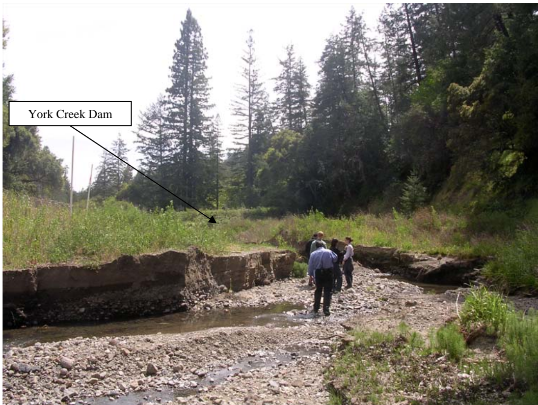
Figure 2. Photo of earthen filled York Creek Dam (looking downstream) (April 8, 2008).
