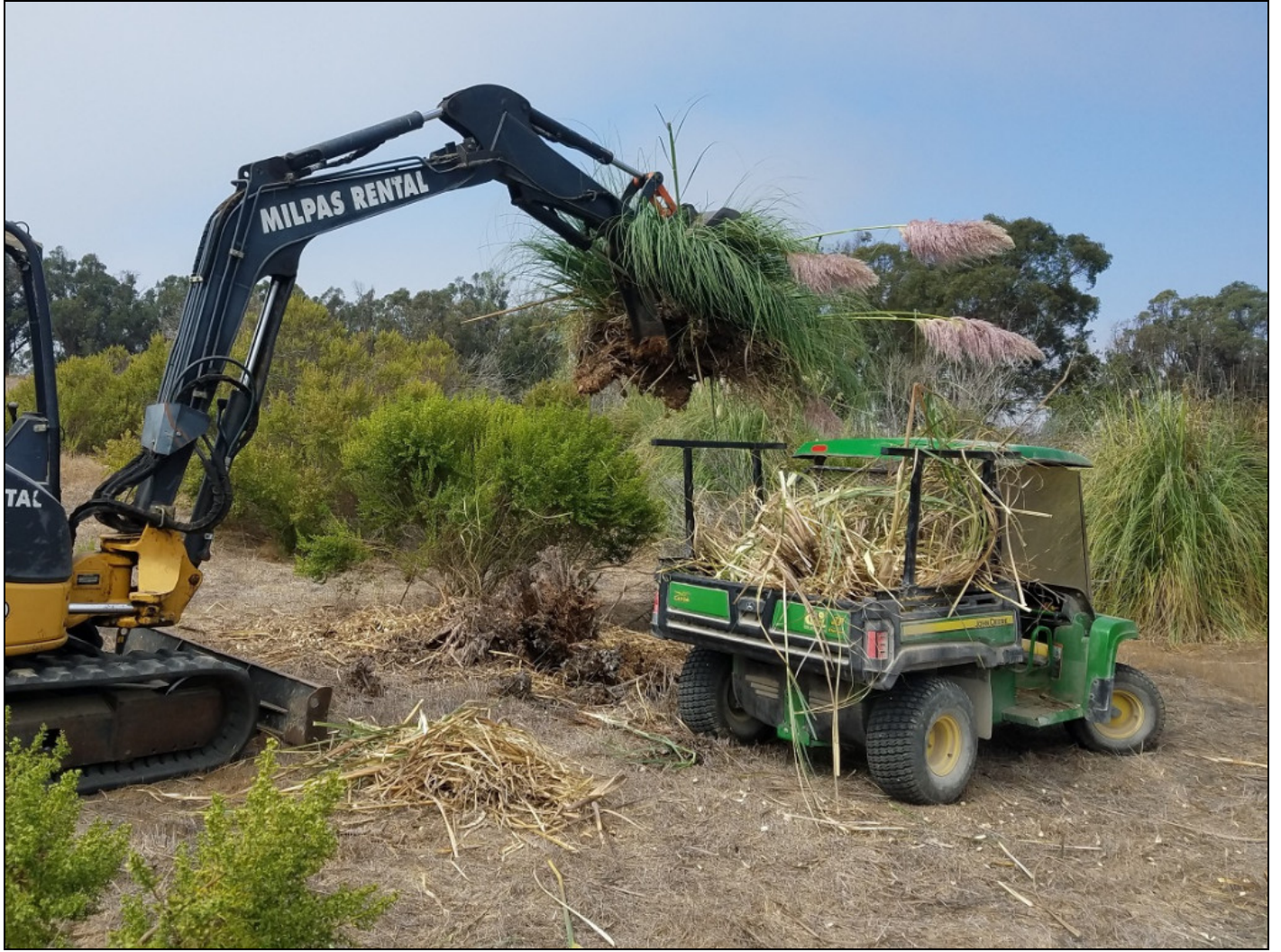
An excavator recently used to help remove Pampas Grass, a large weed that is difficult to remove by hand.
