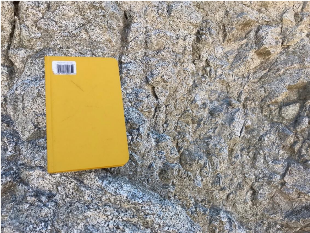
Figure 1.7. Outcrop of the tectonically brecciated basement in foot wall of the proto-Vallecito fault (diagonal lines overlay pattern on map). The rock is shattered but not disarticulated. Yellow field notebook for scale. View azimuth 100 in upper image, 135 in lower image. Photo location available in the appendix.
