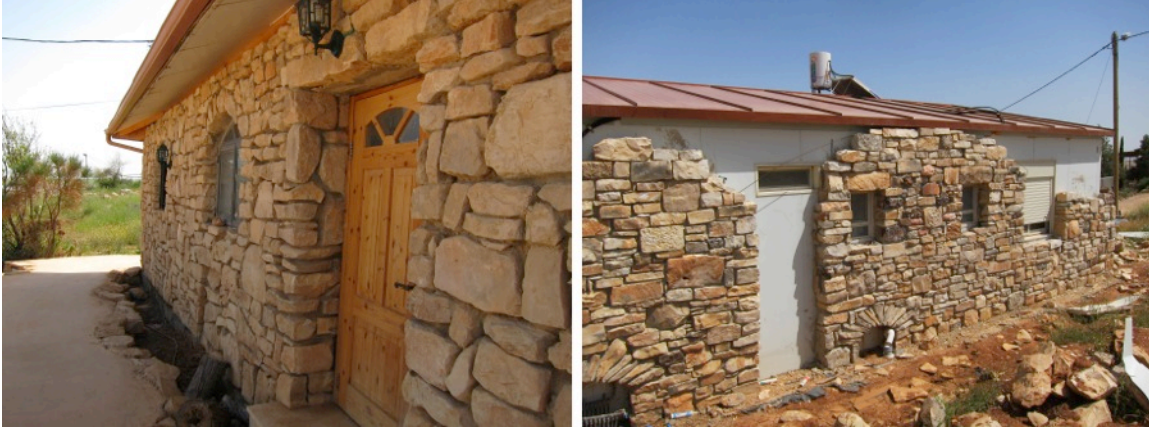
Figure 5.25 Metal-panel-structures covered with a thick layer of stone in the outposts of Tekoa Dalet (left) and Bnei Adam (right). Photo by the author.
