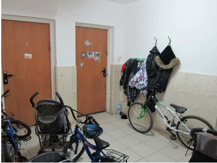
Figure 4.30 Staircase space in Beitar Illit. Those lacking the means to renovate and expand their apartments have often extended their units towards the staircase. They have placed wardrobes and cabinets in the space leading to their apartments. Many also use the shared spaces of the building as storage space for baby strollers and bicycles. Photo by the author.
