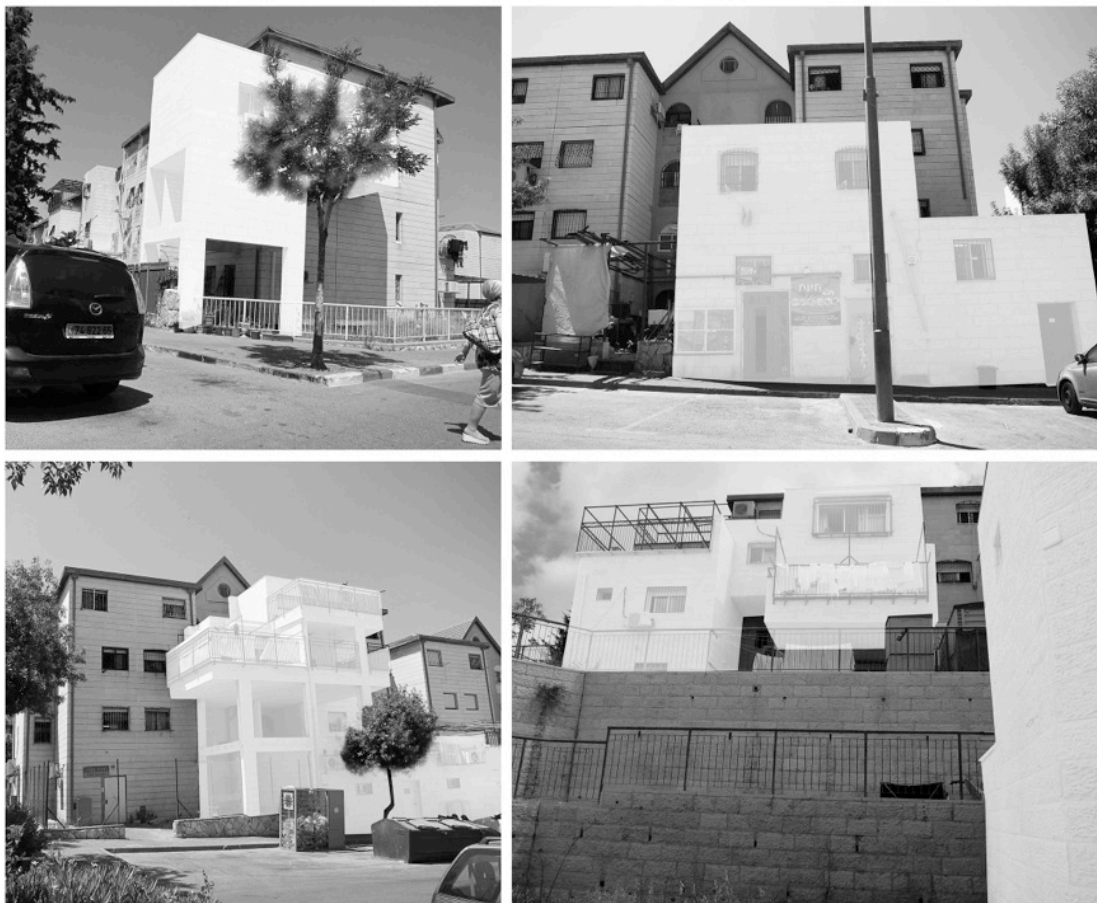
Figure 4.29 Building additions in Beitar Illit. Additions highlighted in white. Beitar Illit, 2015. Photographs by author.
