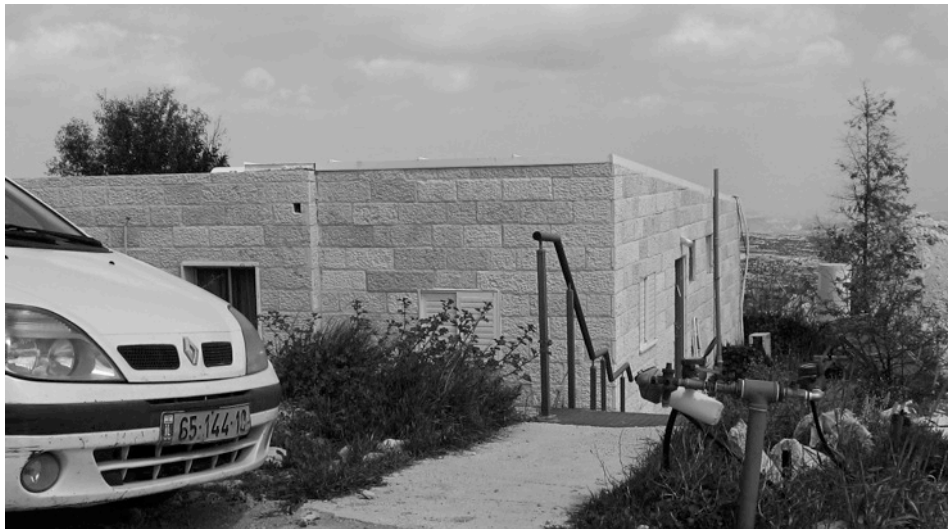
Figure 5.14 The portable placed on top of the covered concrete foundations. After some six months the couple started renovating the portable, they added rooms, a balcony space, and clad it with a thin layer of stone. Later, with time, they added more and more spaces, and today, in addition to their own unit, they have a rental one, all arranged around the original portable. Photo by the author.
