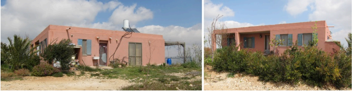
Figure 5.16 Leah and David’s house, 2015. Photos by the author.
