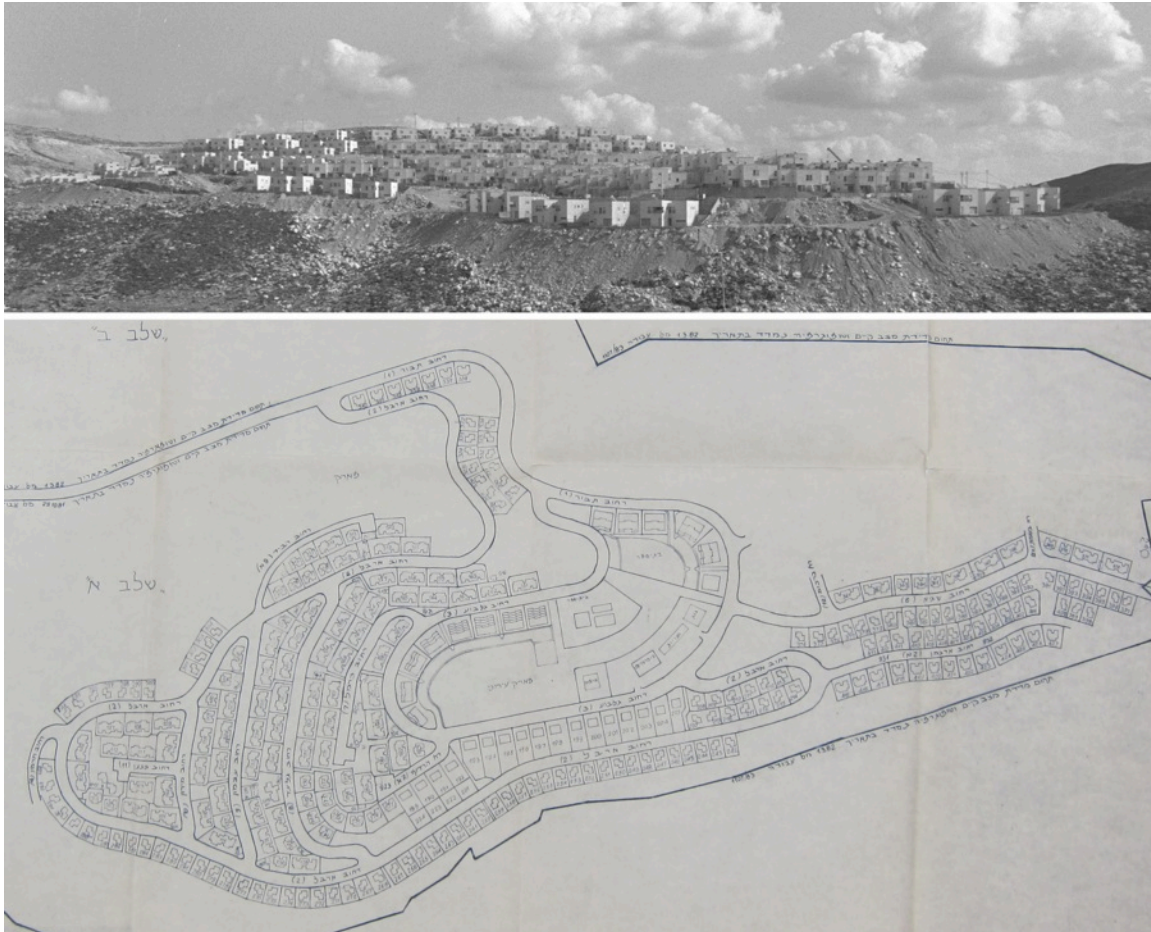
Figure 3.19 Plan of Alfei Menashe from March 1985 (bottom) [ISA] and view of Alfie Menashe (top), 1984. Sources: Israel State Archives and the National Photos Collection of Israel.
