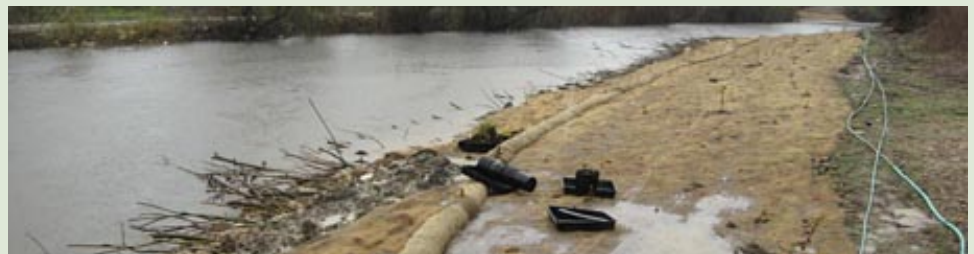
The project handled the first storms of 2008 in fine form, enabling more natural creek processes to occur. This water level reflects a relatively large storm event, likely to occur about once every 5 years
