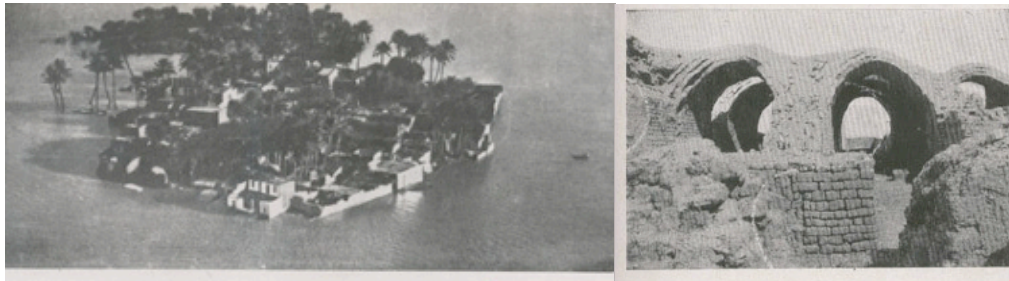
Fig. 1.13, 1.14 The Dilapidating Mud-brick Structures. Source: Harvard University Library PDS, Majallat al-'imārah (1940:1), 216-245, accessed February 28, 2014, http://pds.lib.harvard.edu/pds/view/ .
