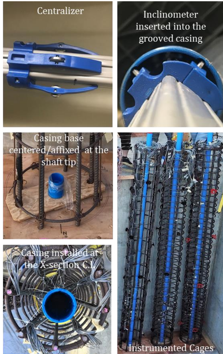
Figure 4-2 Inclinometer setup
