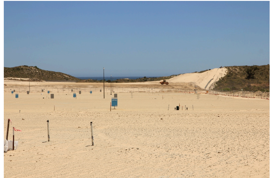
Figure 5. Northern Perth suburb of Alkimos, illustrating the elimination of retaining walls through the total leveling of sand dune topography. The dunes visible in the background originally covered the entire site (author 2014).
