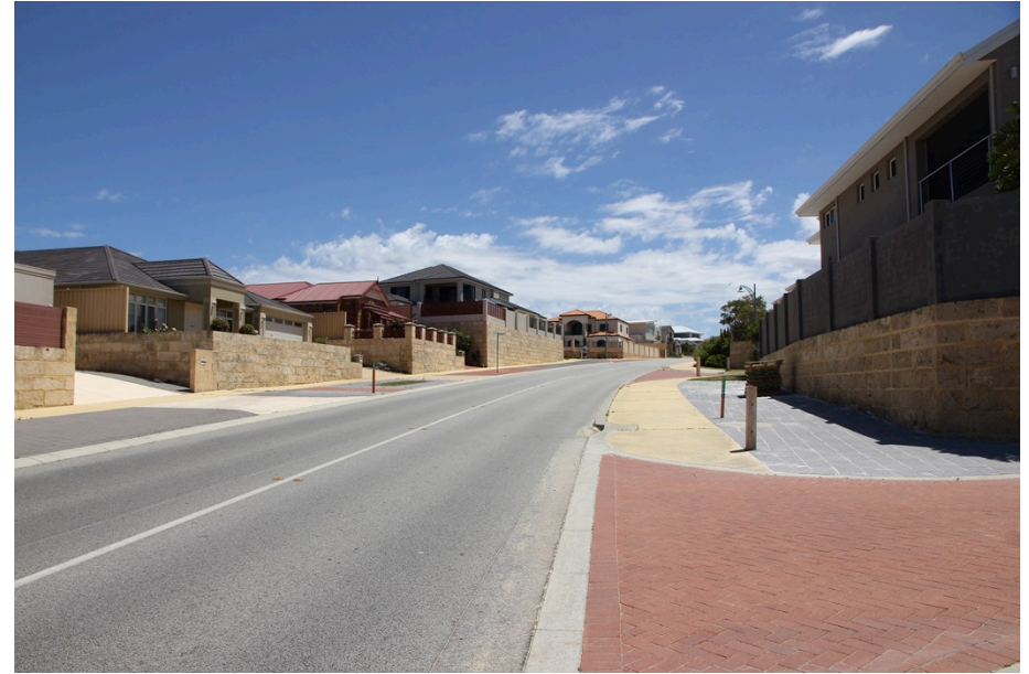
Figure 8. Circa 2010s house set on sand pad that fills out the entire lot and is retained at the property boundaries (author 2014).
