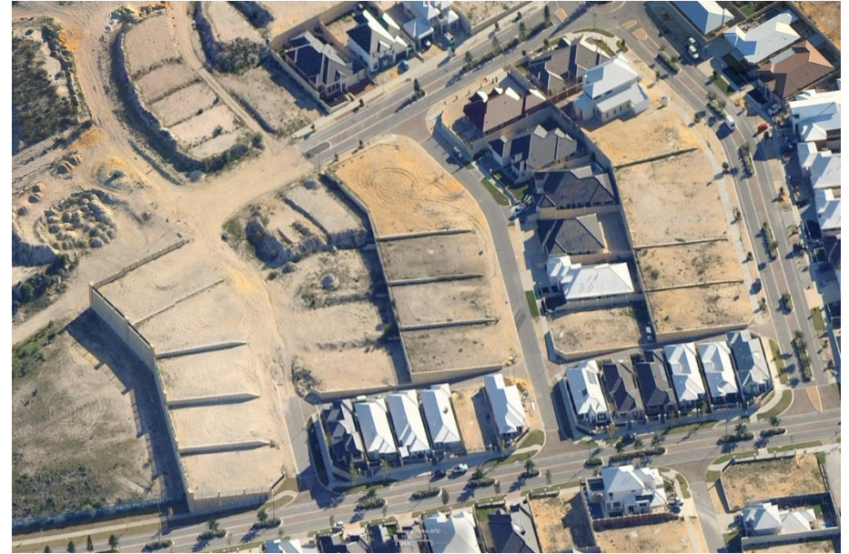
Figure 1. Northern Perth suburb of Jindalee illustrating retaining walls up to 20ft high (© 2012 Google).
