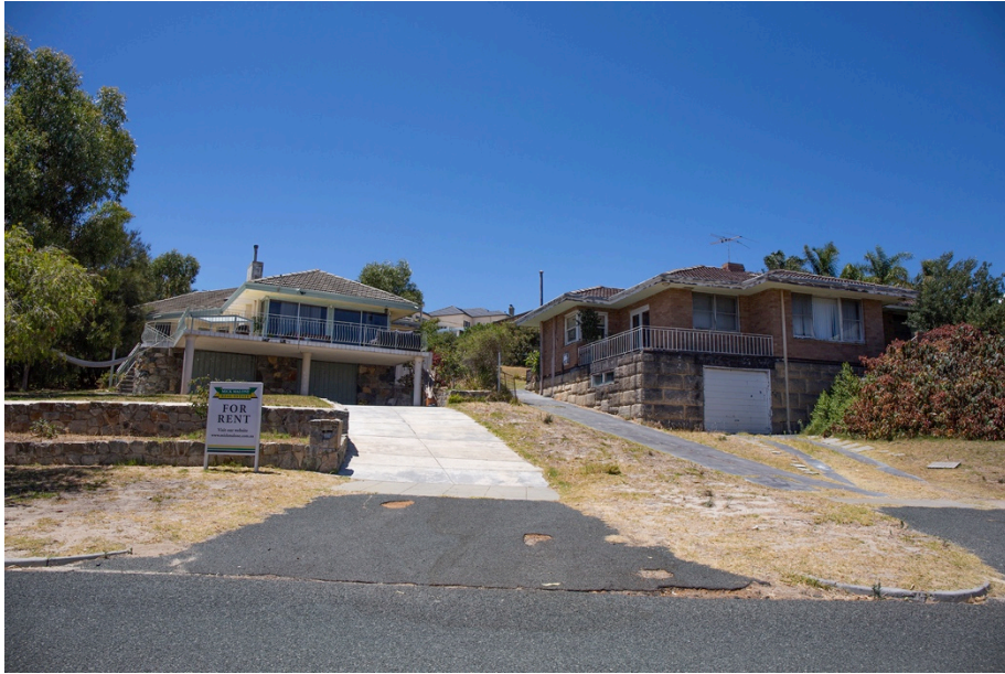
Figure 7. Circa 1950s houses set on limestone plinths that accommodate variations in topography without major earthworks (author 2015).
