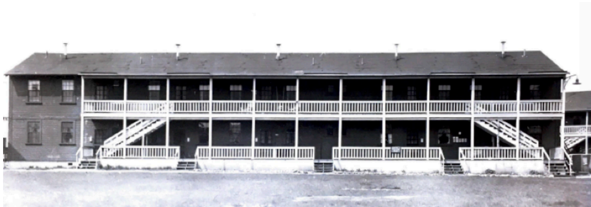
Fig. 2.5 Westgate Apartment Building (Bemis Foundation Papers, Distinctive Collections, Massachusetts Institute of Technology)
