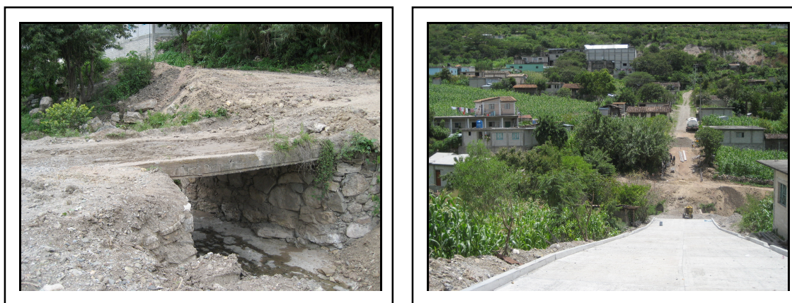
Image 3.1: Bridge in San Miguel Tlacotepec
