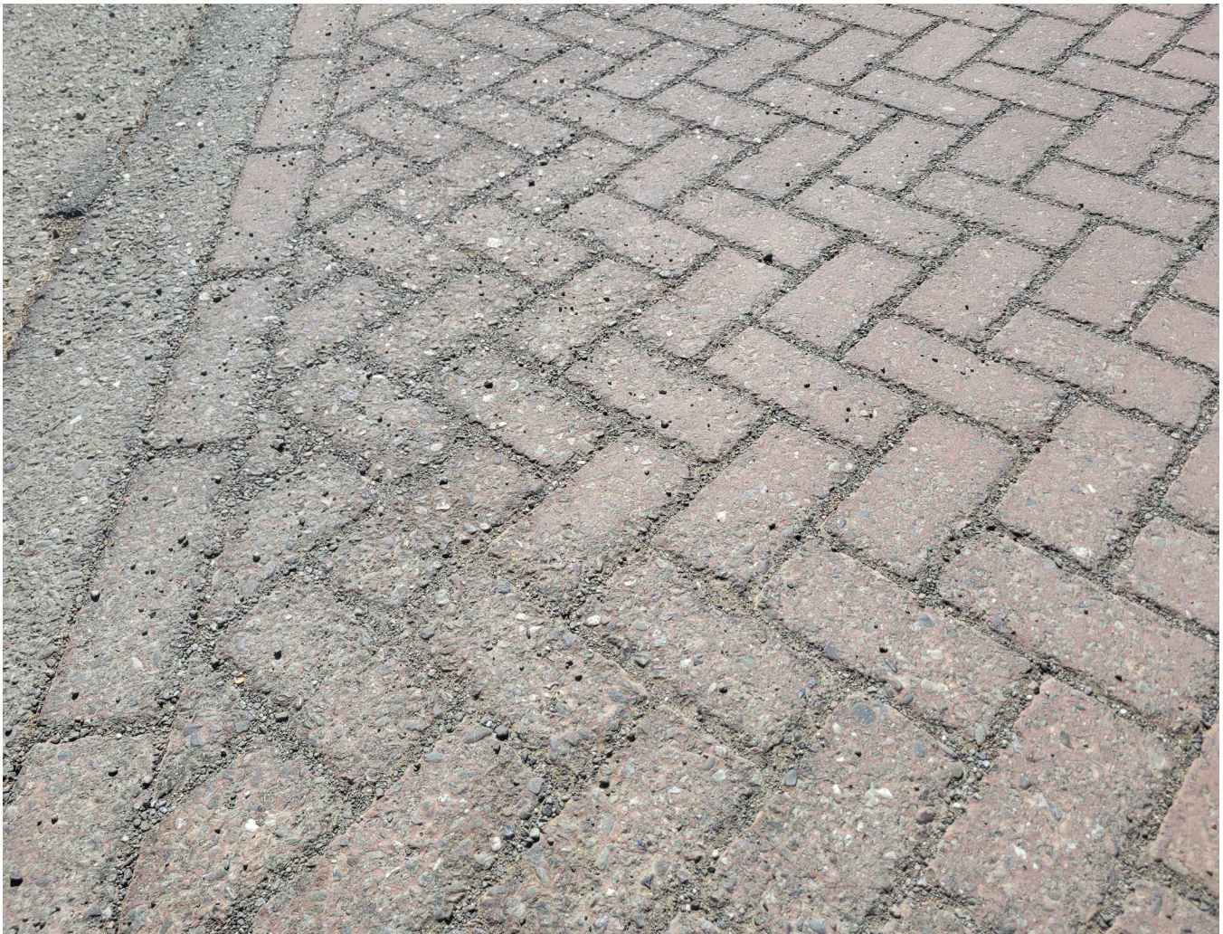
Figure 3.7: Close-up picture of the shoulder showing stamped asphalt in the shape of pavers.
