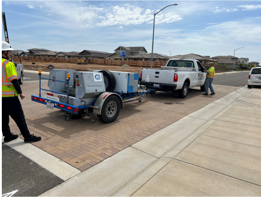
Figure 3.15: FWD testing on the ICP section at an intersection in Rancho Cordova.
