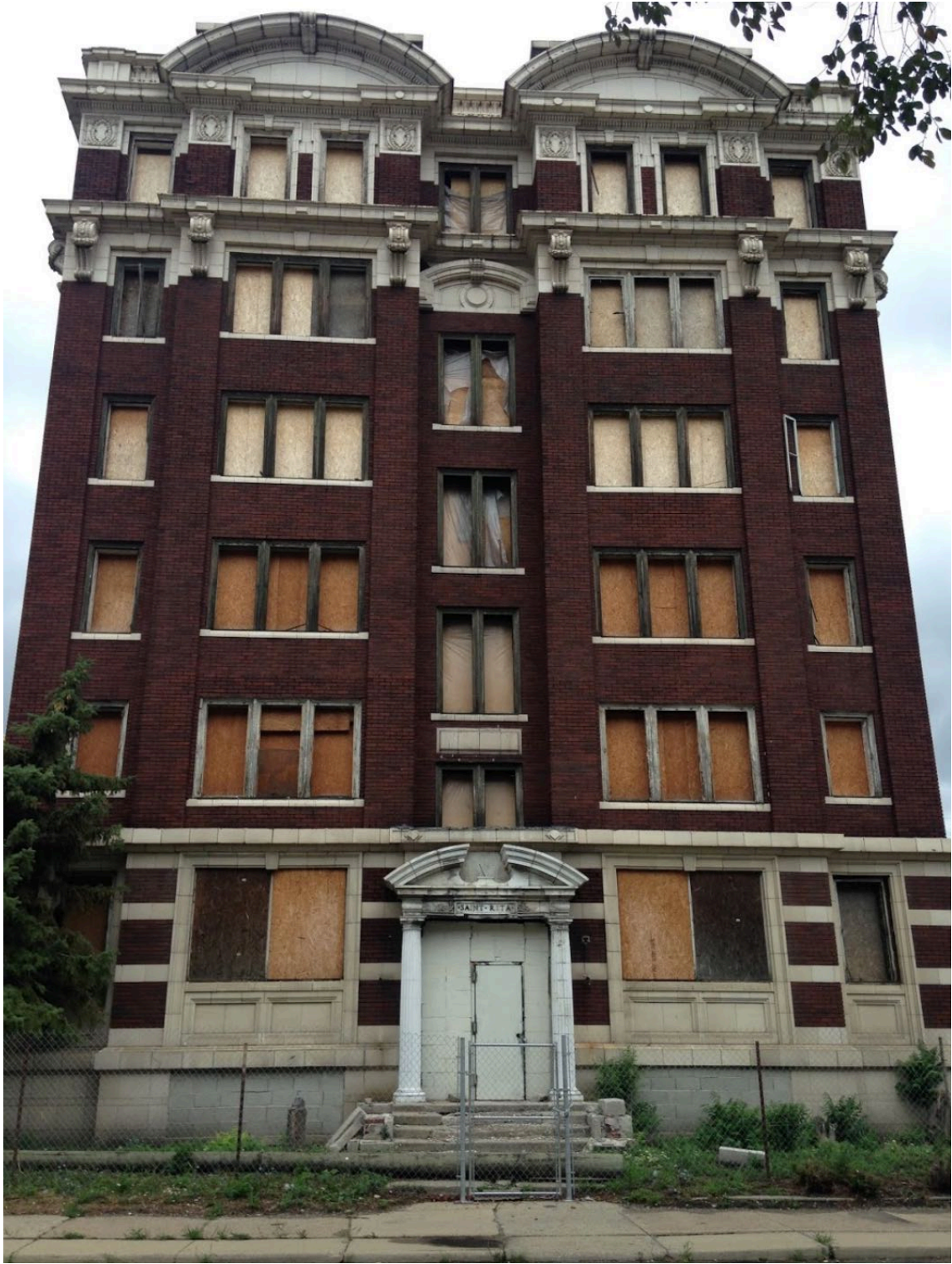
Boarded up windows means someone has plans for this building.
