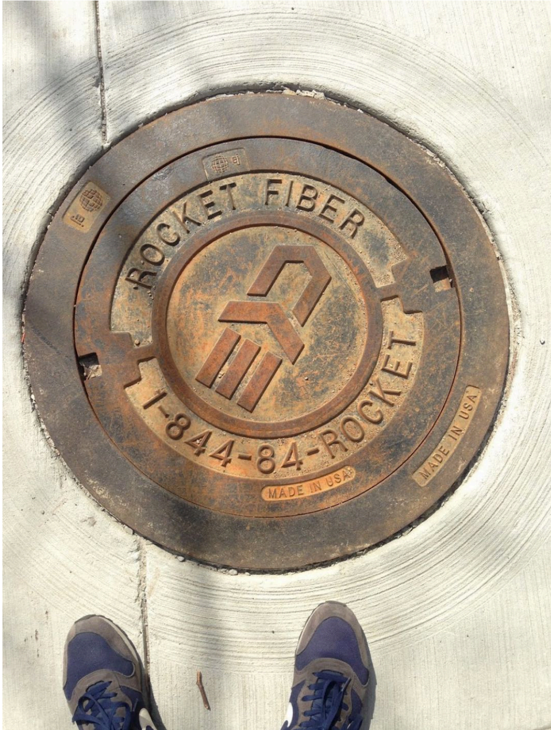
Rocket Fiber manhole cover in mid-town along the Qline.
