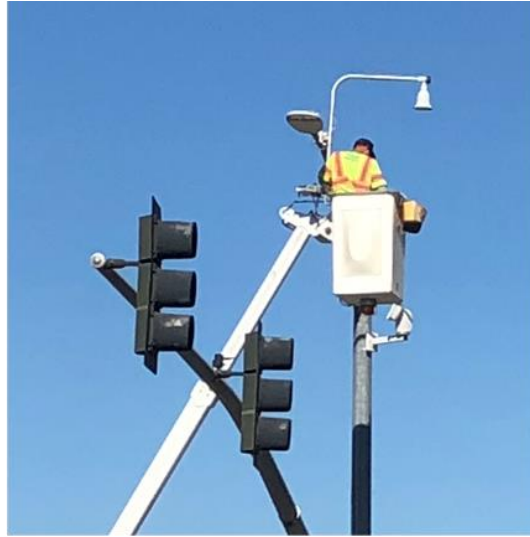
(b) Installing Camera on Street Lamp Post
