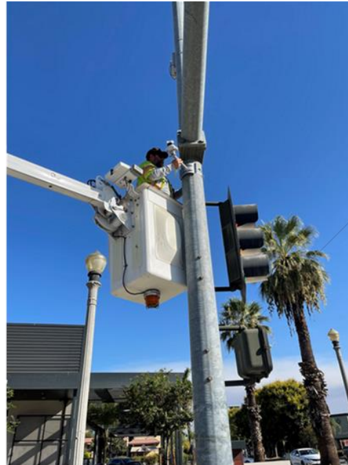
(b) Installing LiDAR on Signal Pole
