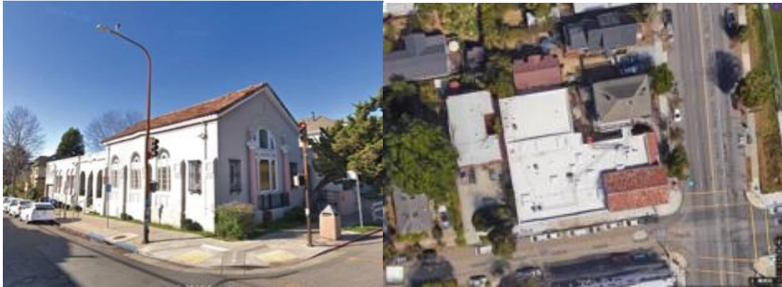
Figure 15. Site Demonstration at City of Berkeley Mental Health Services, 2640 Martin Luther King Jr Way - street view and roof layout
