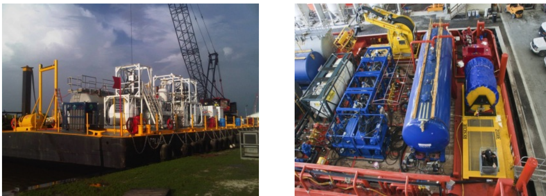
Figure 3.6: Two BPWS Integrated Systems installed on the D&L Salvage barge The Splash (left) and four BPWS Integrated Systems installed on the Edison Chouest platform supply vessel ELLA G (right). Images courtesy of Professor Eric Hoek, UCLA.
