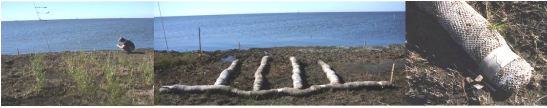
Figure 3.10: Shoreline restoration studies conducted in Bay Jimmy; transplant plot (left); propagation tube plot (center); detail of propagation tube (right).
