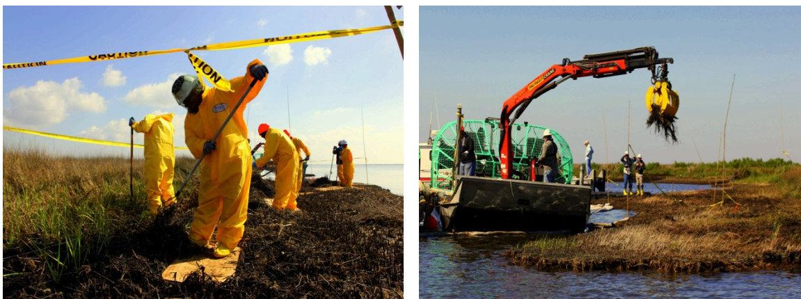
Figure 3.3: Aggressive remediation of oiled shoreline in Bay Jimmy (Barataria Bay, Louisiana). Cleanup crews manually raking oiled debris and cutting oiled vegetation (left); mechanical removal of oiled material (right). Photos courtesy of P.J. Hahn.
