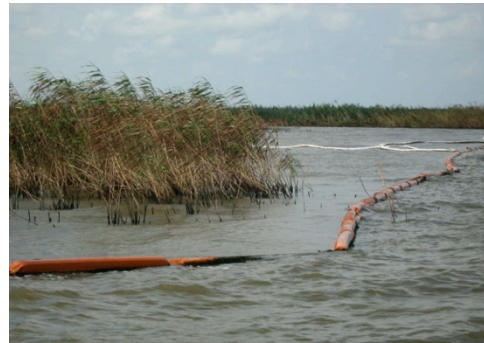
Figure 2.4: Oil containment boom deployed as a temporary protective barrier. Image courtesy of Andy Nyman, Louisiana State University.
