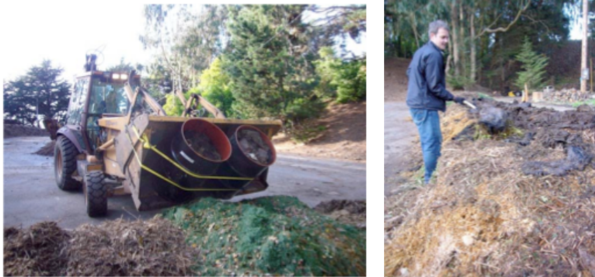
Figure 4.1: Presidio remediation project. Adding oil-contaminated hair mats to green-waste compost for the start of the bioremediation process (left). Distributing the hair mats in preparation for thermophilic composting (right).
