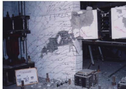
c. 8 th Floor coupling beam (3.85% drift)
