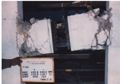
b. 8 th Floor coupling beam (3.33% drift)
