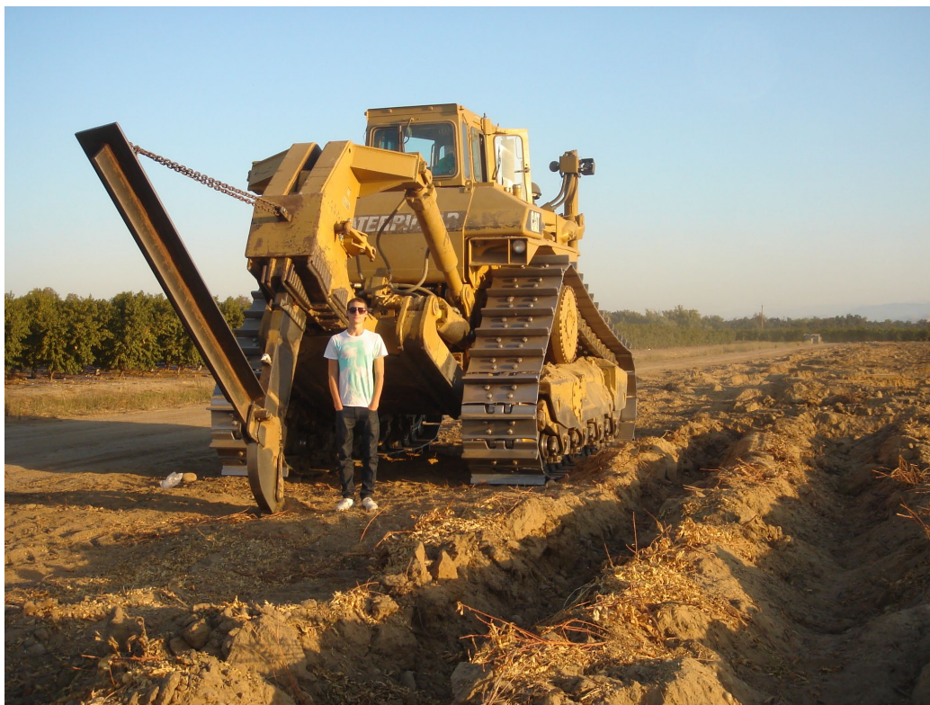
Figure 4-4. Showing Slip Plow Used to Loosen Deep Soil Layers.
