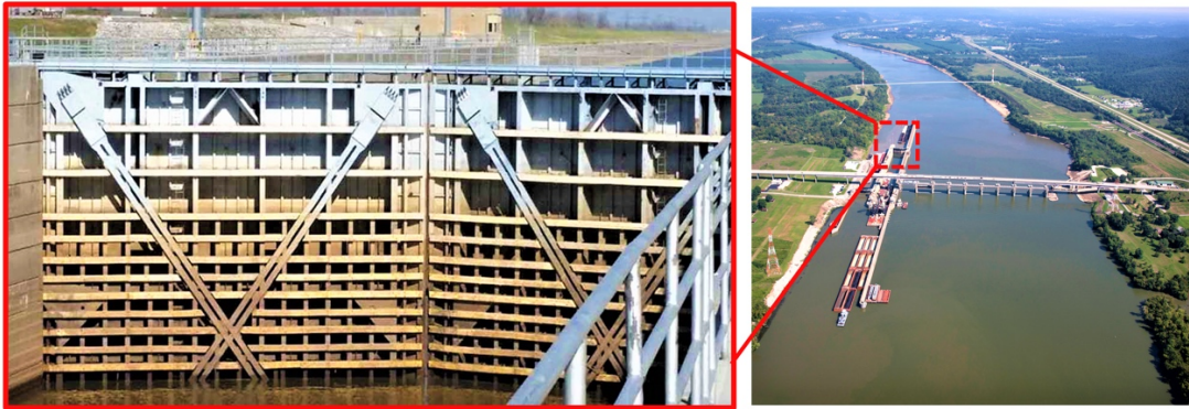
Figure 3.1: Greenup locks and miter gate
