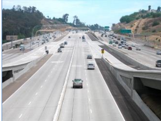
Figure 4-3 – I-15 Express Lanes at Rancho Bernardo Direct Access Ramp Overpass
