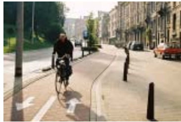
Bicycle Lane in Leuven, Belgium. Lane is near sidewalk-grade and separated from the street
