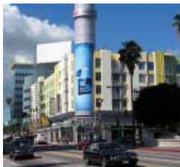
Figure 13: Sunset and Vine features ground floor retail with housing above
