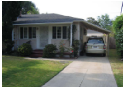
Figure 5. Private gate to second unit behind main house.
