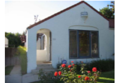
Figure 8. Front of main house (east elevation)
