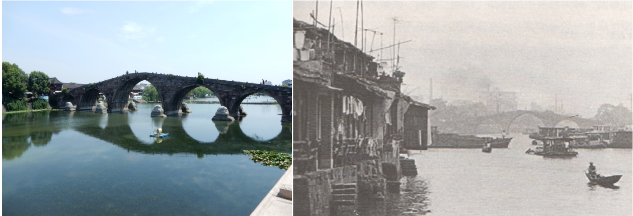
Figure 2- 7: Guangji Bridge now and then. (Left) Photography by the author; (Right) From Lao (2015, p. 27).
