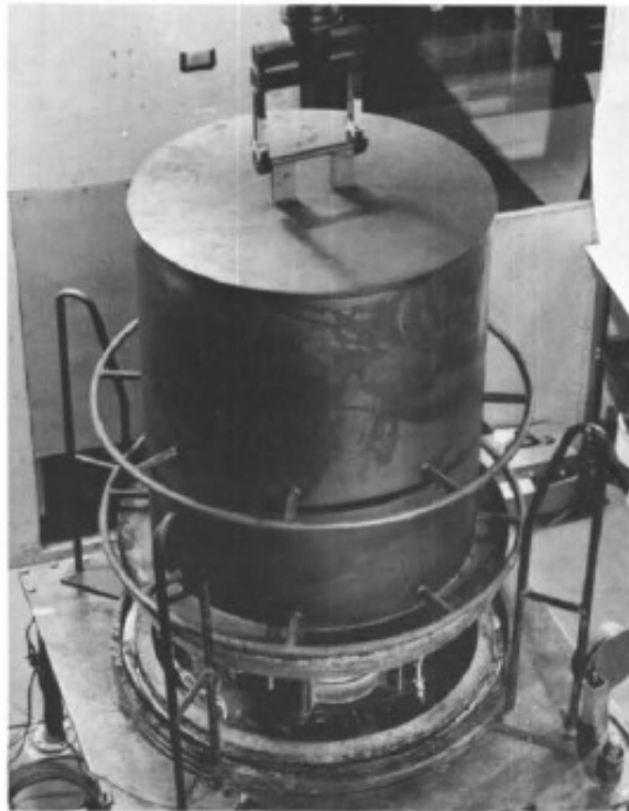
Figure 2.12: Melt refining furnace [5]
