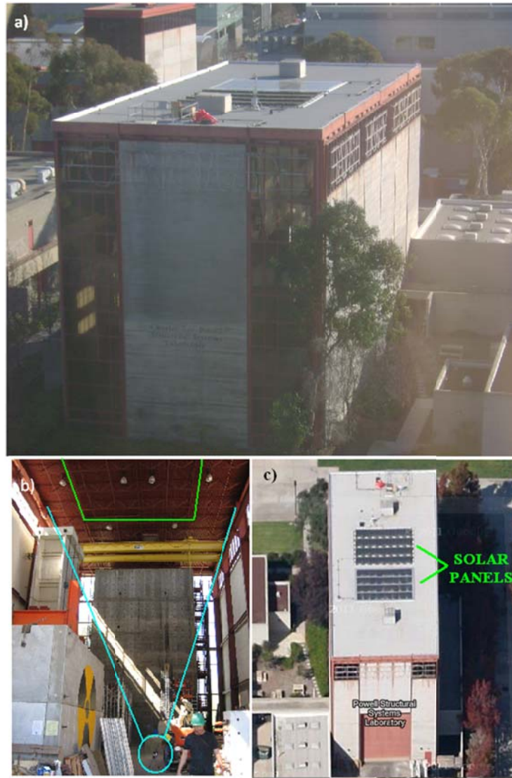
Fig. 1. a. Photograph of PoSL facing South; b. Photograph of PoSL from inside facing North with TIR camera circled, field of view shown by blue lines, and PV location outlined in green; c. Google Earth image of PoSL (North is up) with tilted array on the North side of the roof and
