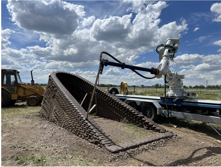
Figure 7.13: 3D-printed Nubian vault during the construction phase.
