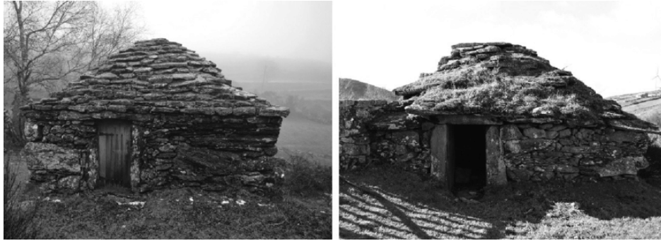
Figure 7.1: Cardenha buildings in Vale de Poldros featuring corbelled masonry roofs [71].
