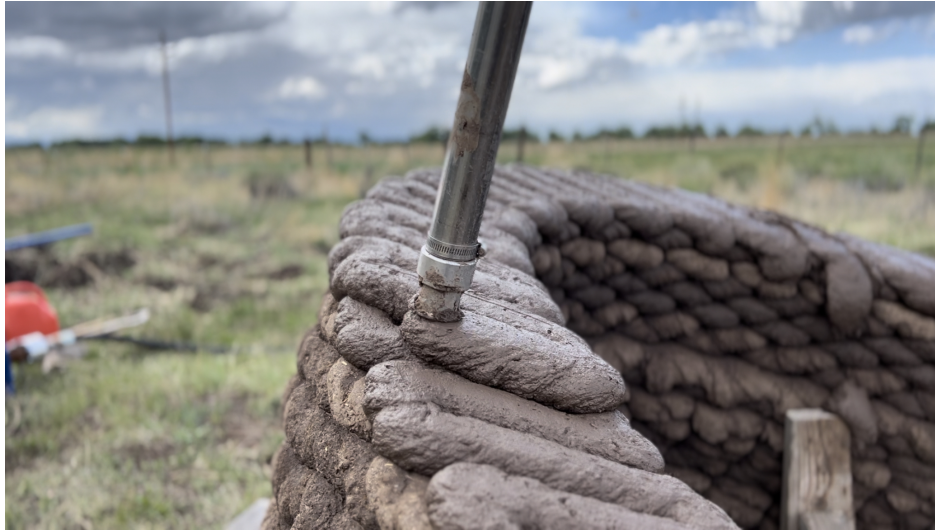
Figure 7.12: 3D-printed adobe following a square-wave toolpath pattern.
