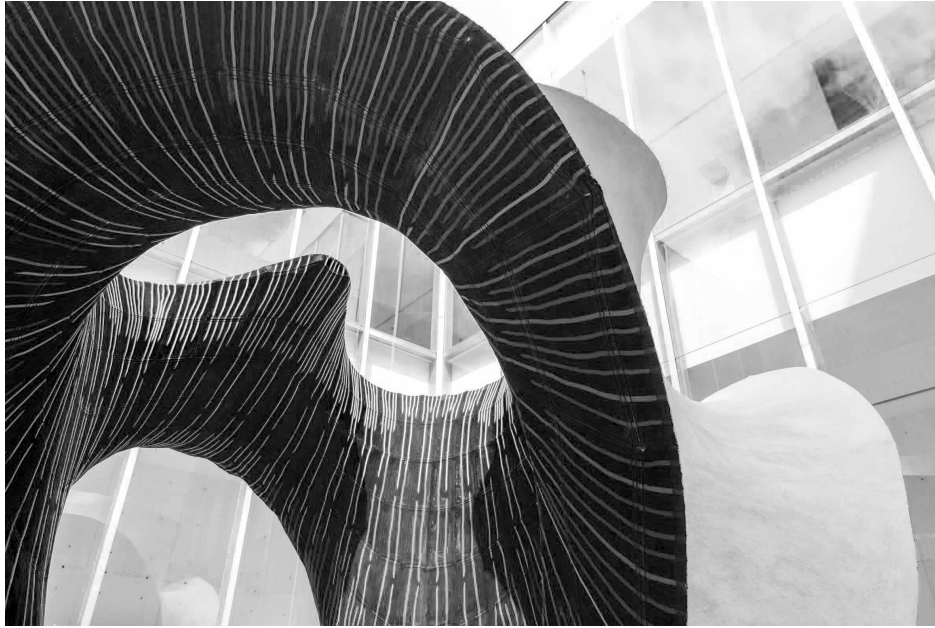
Figure 2.12: KnitCandela, a sinuous concrete shell built on an ultra-lightweight knitted formwork [232]
