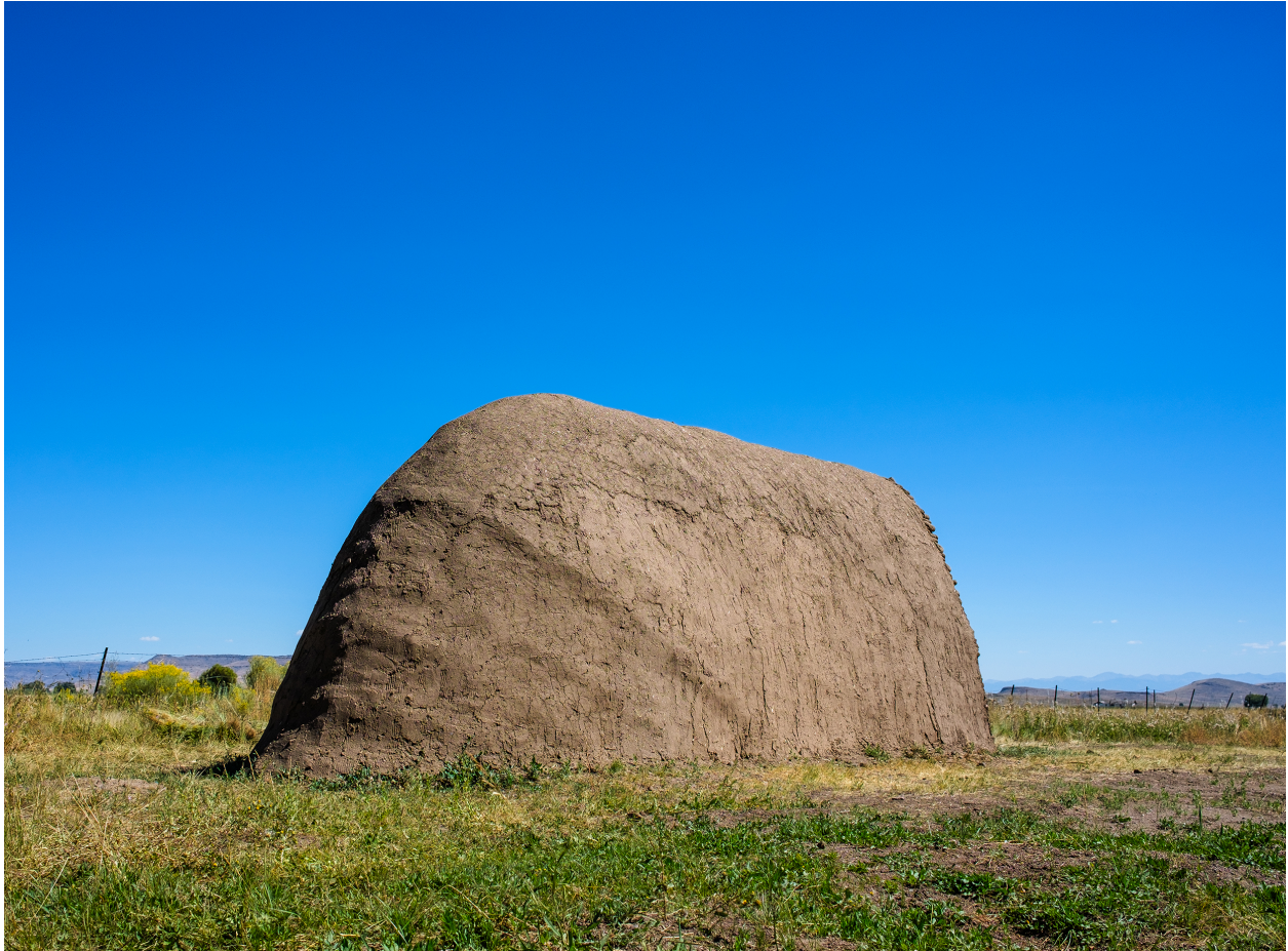
Figure 7.15: The 3D-printed Nubian vault after plastering the outer surface with adobe.
