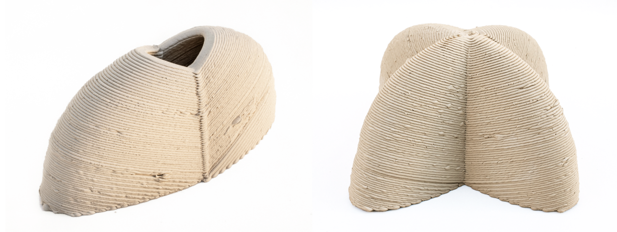
Figure 7.9: Intersecting Nubian vaults built using clay 3D printing.
