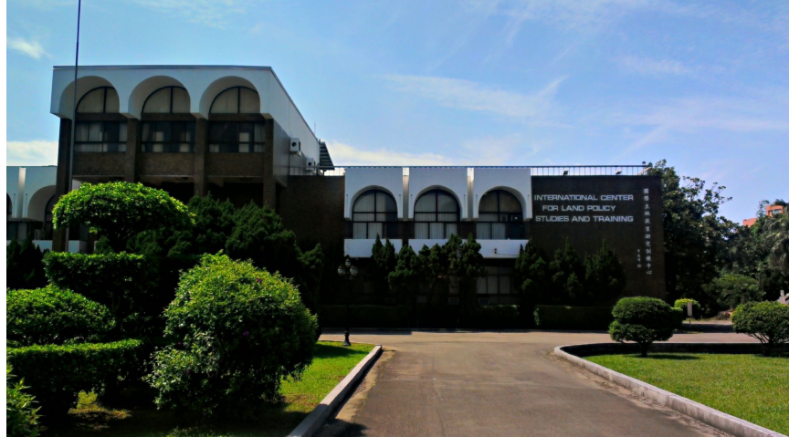
Photograph: The Land Reform Training Institute building in Taoyuan, Taiwan, which was renamed the International Center for Land Policy Studies and Training in 2000. Picture taken by author in 2013.
