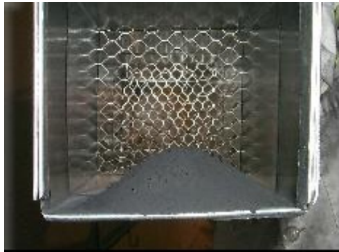
Figure D2. Dust deposited below the injection site
