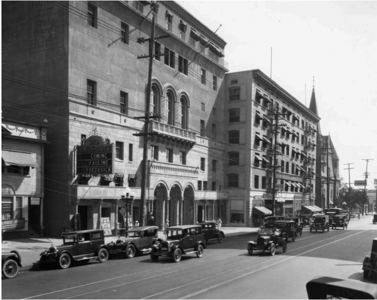
Figure 1.21: View of the FMC in context, 1926. Source: Los Angeles Public Library, Security Pacific National Bank Collection.
