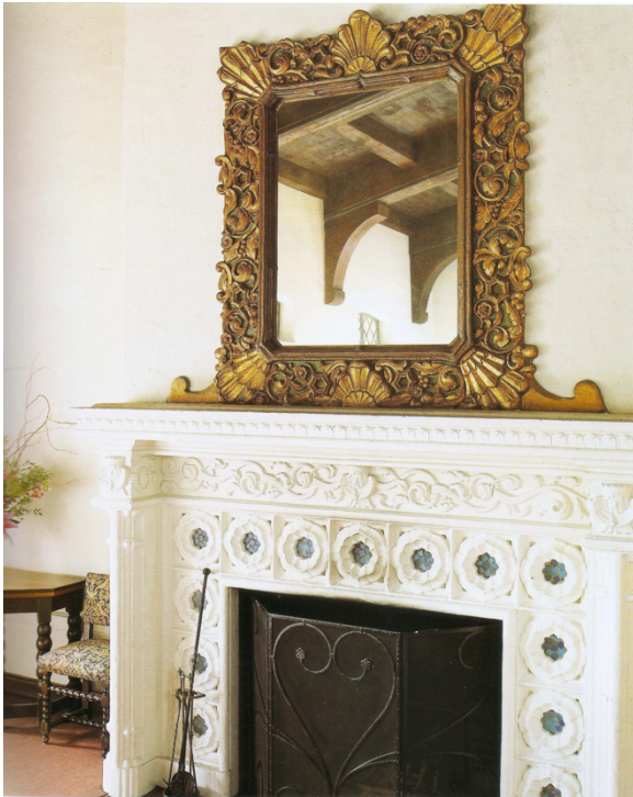
Figure 3.26: The cast concrete fireplace in the BWCC dining room. Note the mirror above reflecting the reinforced concrete ceiling. Source: Mark A. Wilson, Julia Morgan: Architect of Beauty (Salt Lake City, Utah: Gibbs Smith, 2007).
