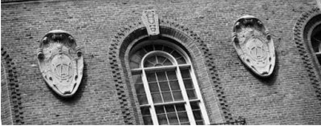
Figure 2.13: The spandrels of central arch on the fourth floor with cartouches depicting the logo and WAC initials. Source: The Metropolitan Club Archives.
