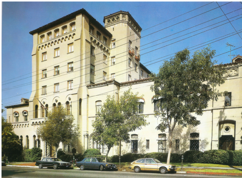
Figure 3.7: The BWCC building. Source: Sara Holmes Boutelle, Julia Morgan, Architect (New York: Abbeville Press, 1988).
