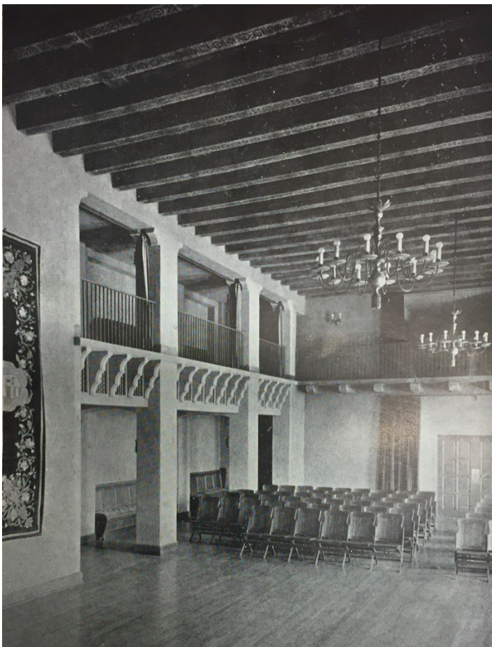
Figure 1.33: FMC third floor lecture or recital hall with painted concrete piers, 1924. Source: "A New Club Building in Southern California," The Architect and Engineer .
