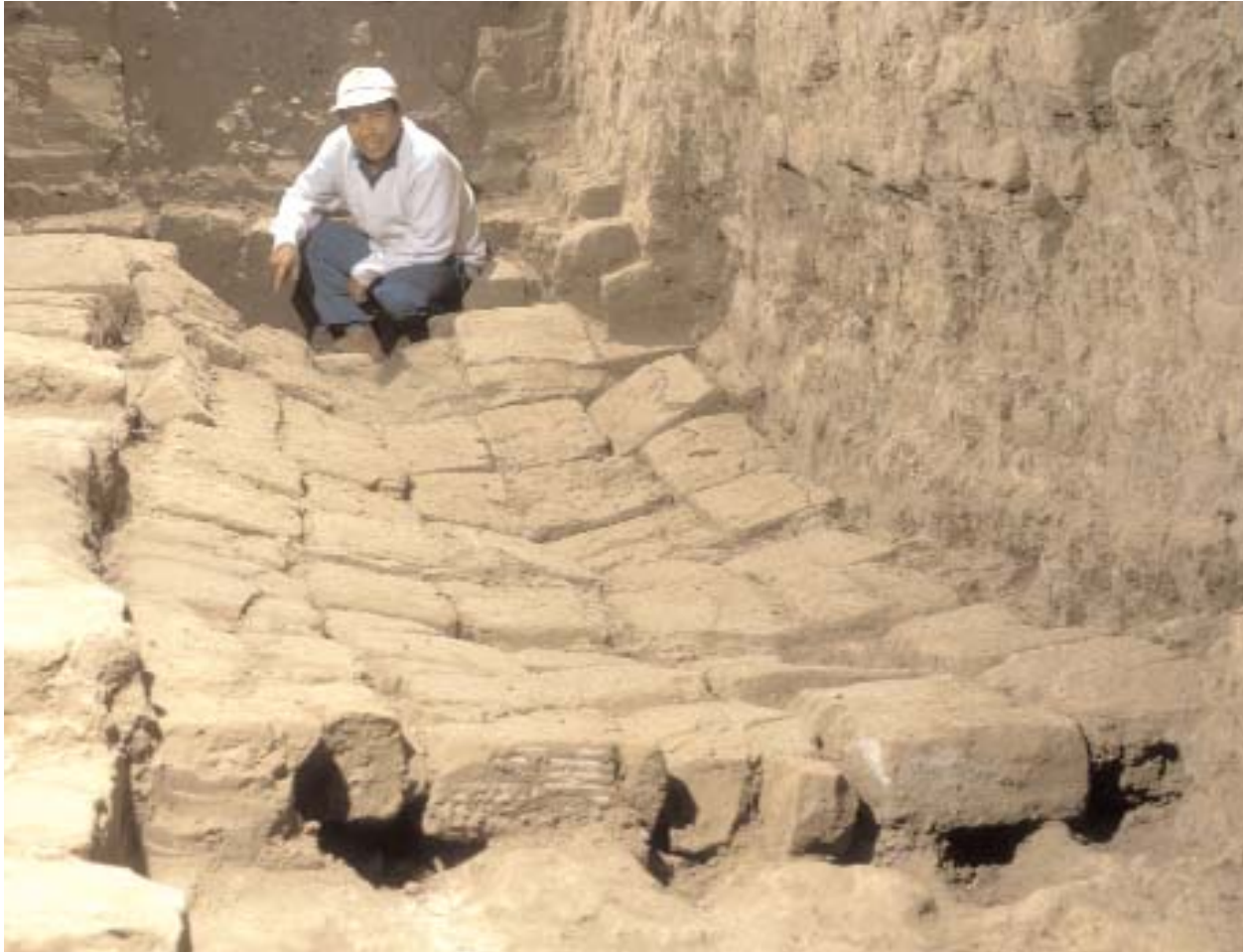
Figure 5.4 The layer of adobes on top of the roof beams. Note the impressions of the decomposed roof beams under the adobes in the foreground.
