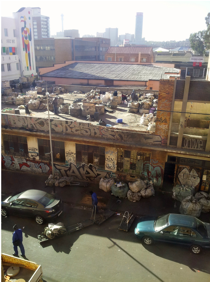
Figure 13. Recyclers' Building, Fox Street. Source: Author's Photograph, 2014.
