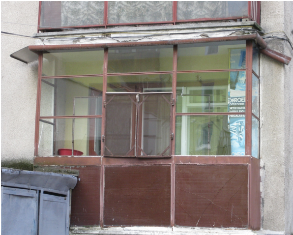
Fig. 9 Balcony enclosure in the Grigorescu neighborhood of Cluj-Napoca, Romania. This image shows the balcony enclosure as was built before 1989. Photo by author, 2011.
