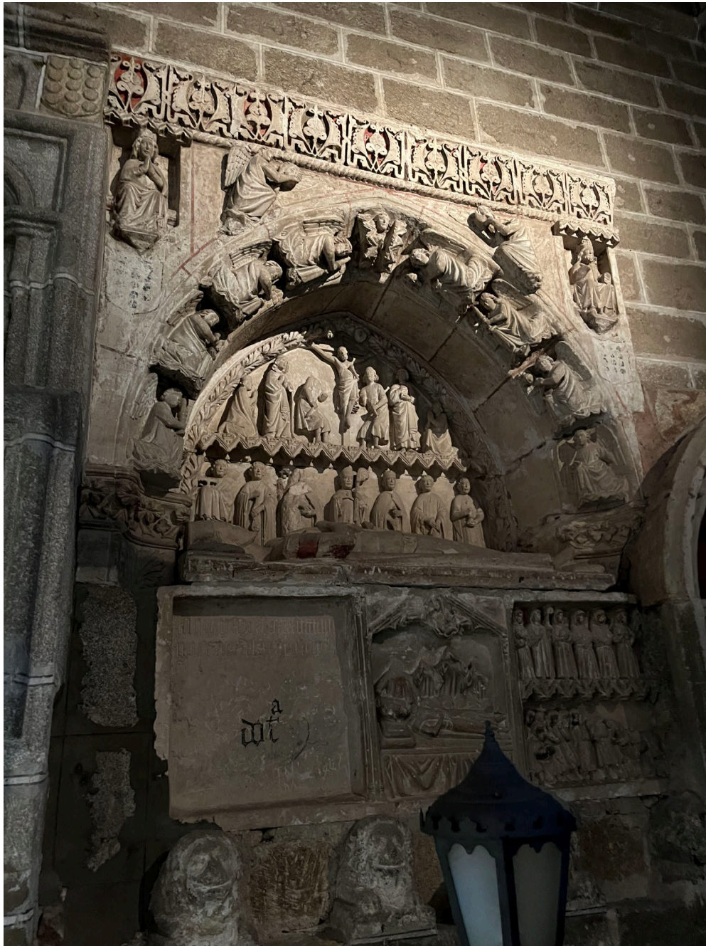
Figure 50: Family chapel of Esteban Domingo in the north tower base, San Miguel chapel Photo: Teresa Martínez Martínez
