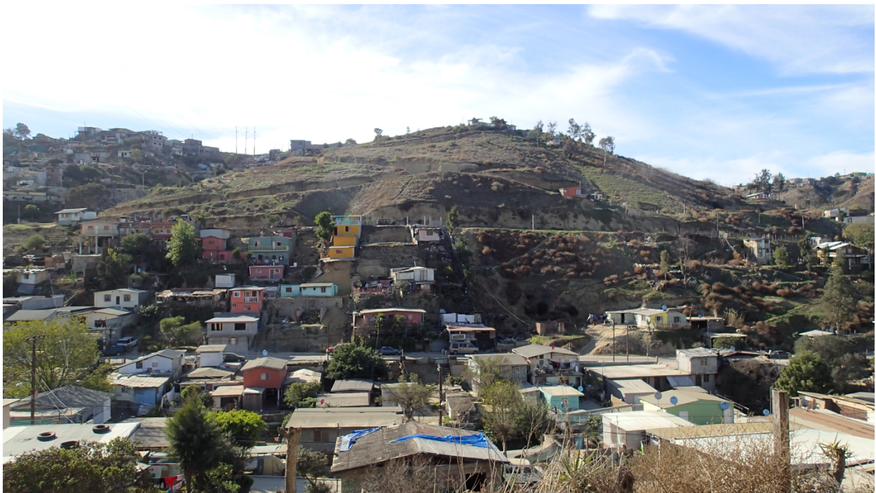
Figure 13. Photo of Divina showing informal development on steep slopes where erodible soil is visible and comprise the foundation of many homes. Source: Photo courtesy of UCSD Center on Global Justice.
