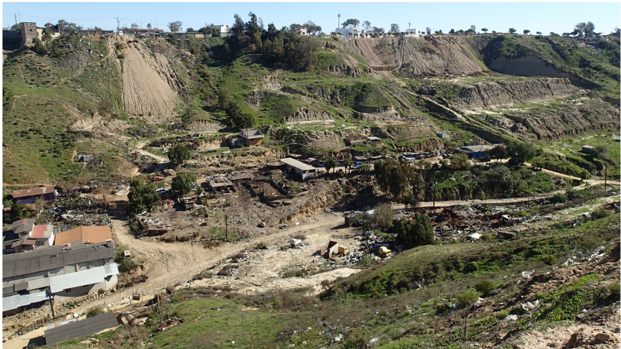
Figure 14. Photo of Alacrán showcasing prevalence of trash in the canyon, deep erosion cuts, and other signs of informal development. Source: Photo courtesy of UCSD Center on Global Justice.
